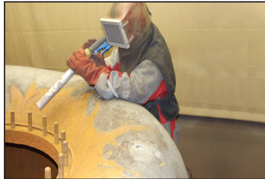
Thorough surface preparation
